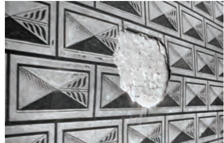
Example of sgraffito in Prague (with patch missing to show plastering)
