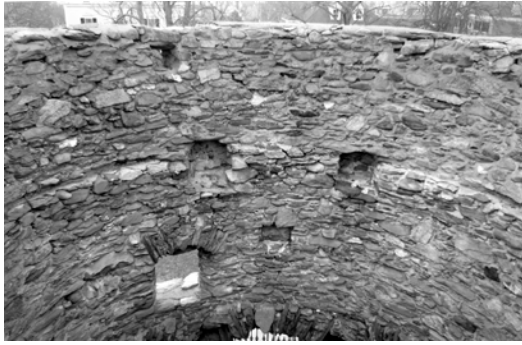
Looking west, the two other beam sockets and the "running mortise" are clearly visible
