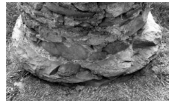
About 1 foot of the drums is buried underground, leaving only about 6 inches visible
