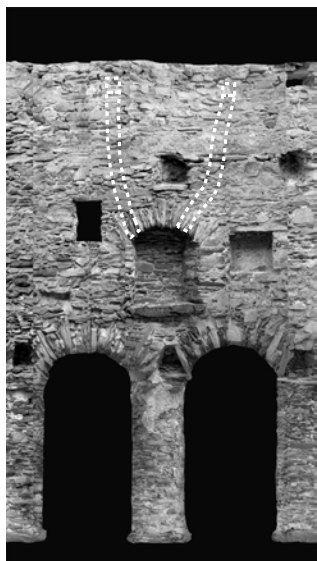
Interior of the Tower, showing where the 2 flues run through the middle of the thick wall
