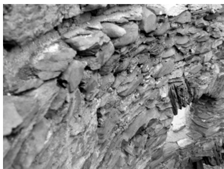
close-up view of the “running mortise” on the southeast part of the interior
